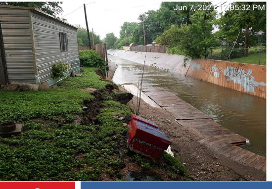
Exhibit shows Bermuda Ditch (West) area retaining wall collapse.
