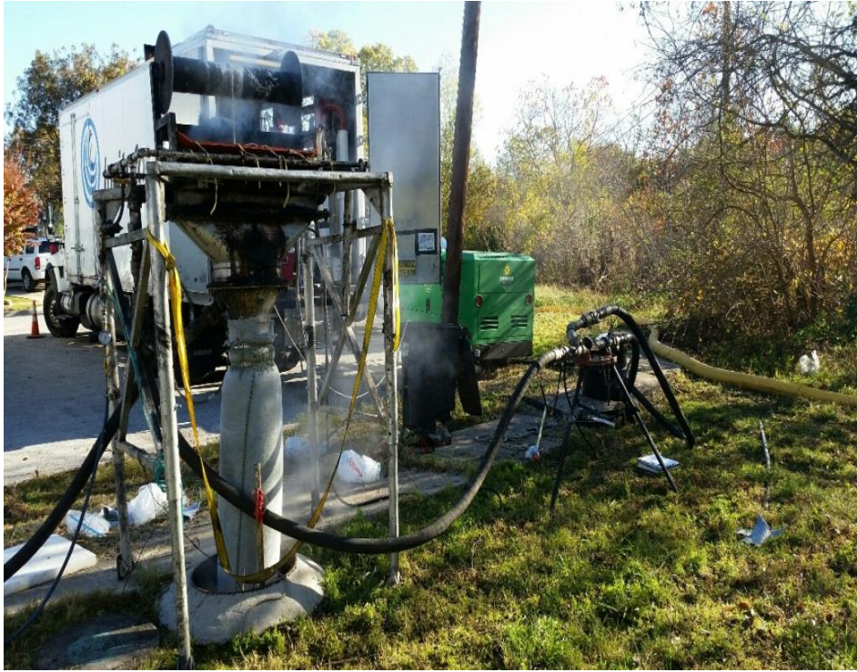
12" Sewer Line Rehab
