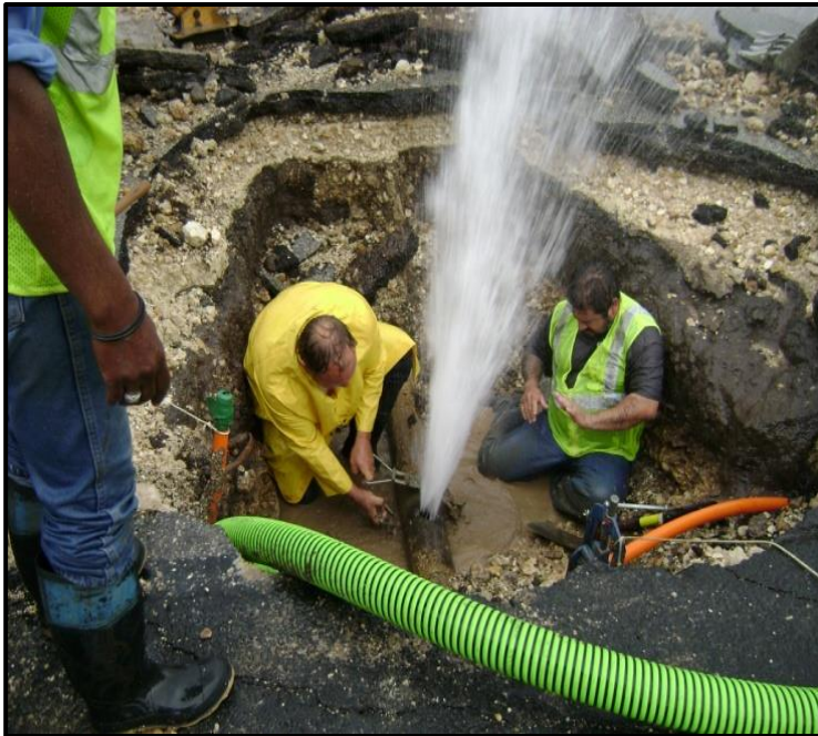
Water Line Rehab Phase 1
