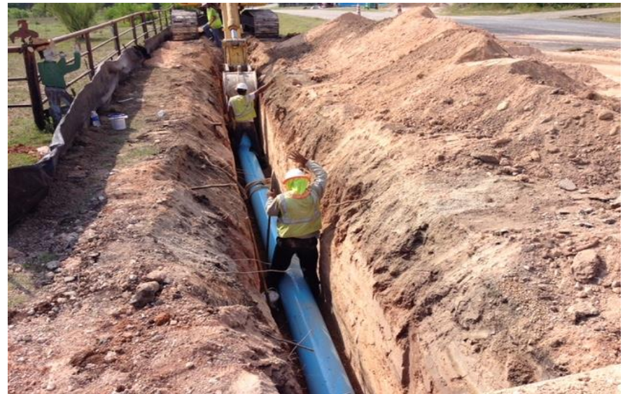
Onion Road Water Line
