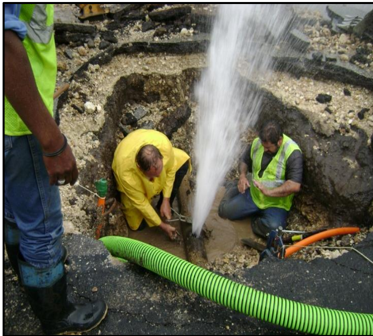
Water Line Rehab Phase 1
