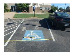
Smart level measuring the slope of an accessible parking space.
