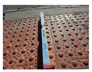
Measuring the slope of a sidewalk ramp.
