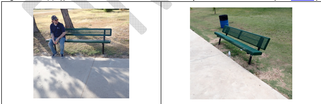
Figure 3.3.1.2(c) Typical Observation: Benches do not have adjacent accessible surface. [TAS 802.1.2. ]
