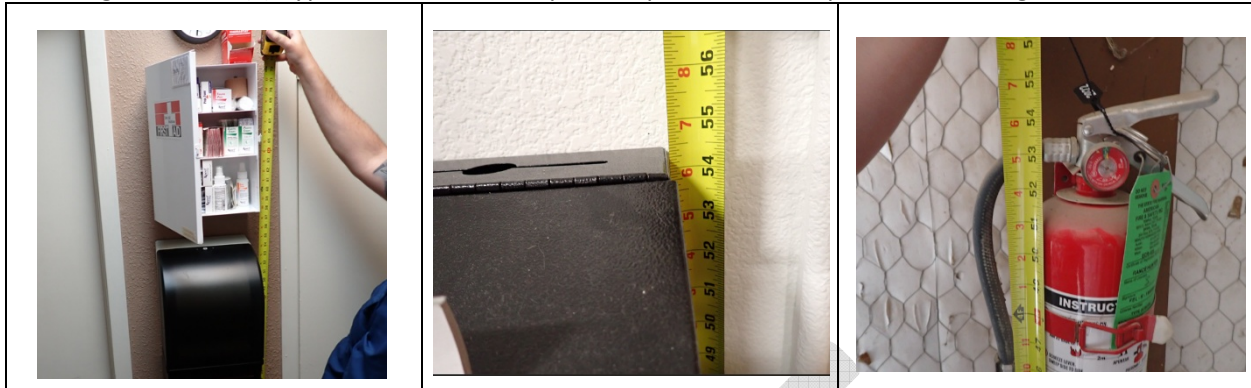
Figure 3.2.1.1(c) Typical Observation: Operable parts above required reach range: [TAS 308. ]
