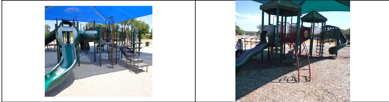
Figure 3.3.1.3(d) Typical Observation: Play area has no ground level play components on an accessible route. [TAS 240.2.1.1 ]
