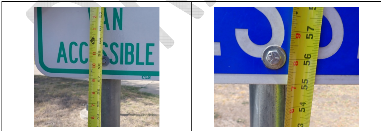
Figure 3.3.1.1(b) Typical Observation: Accessible signs are too low. [TAS 502.6 .]
