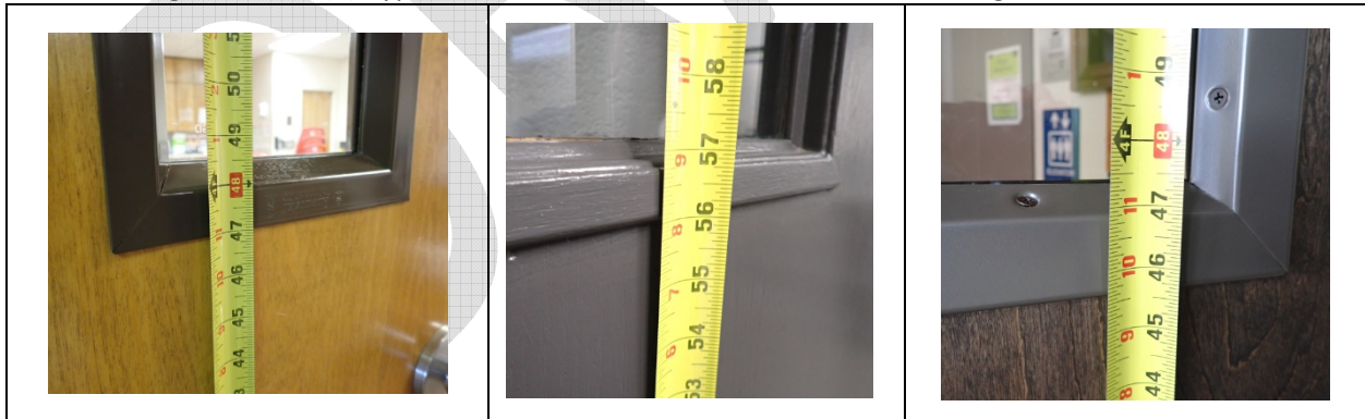
Figure 3.2.1.2(e) Typical Observation: Door vision windows too high: [TAS 404.2.11 ]
