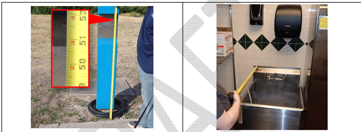
Figure 3.3.1.1(a) Typical Observation: Elements too far or too high. [ADA Standards 308.3.2 ]
