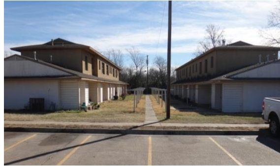
Existing Units at Moss Rose
