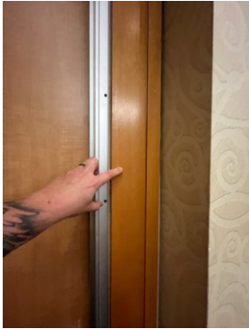
Example of door frames to be painted
