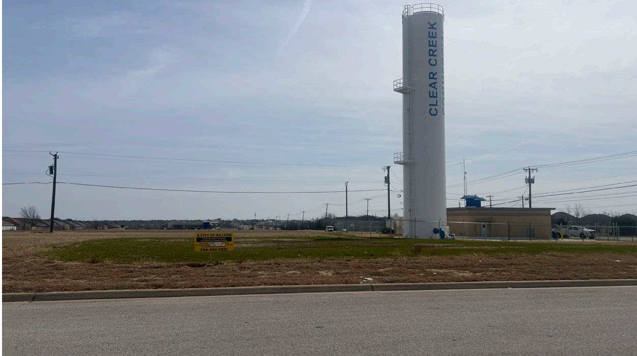
View facing the subject properties from Dayton Drive:
