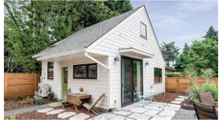
Tiny house on slab
