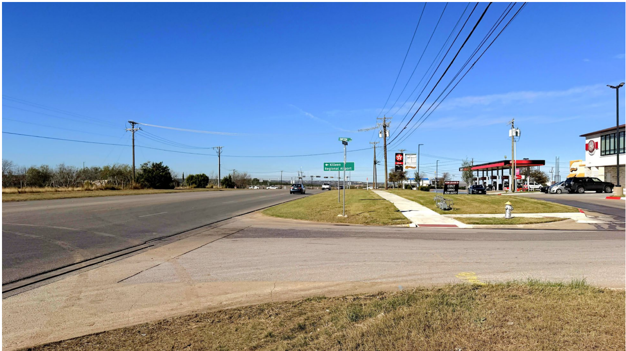
View facing west on West Stan Schlueter Loop towards Clear Creek Road:
