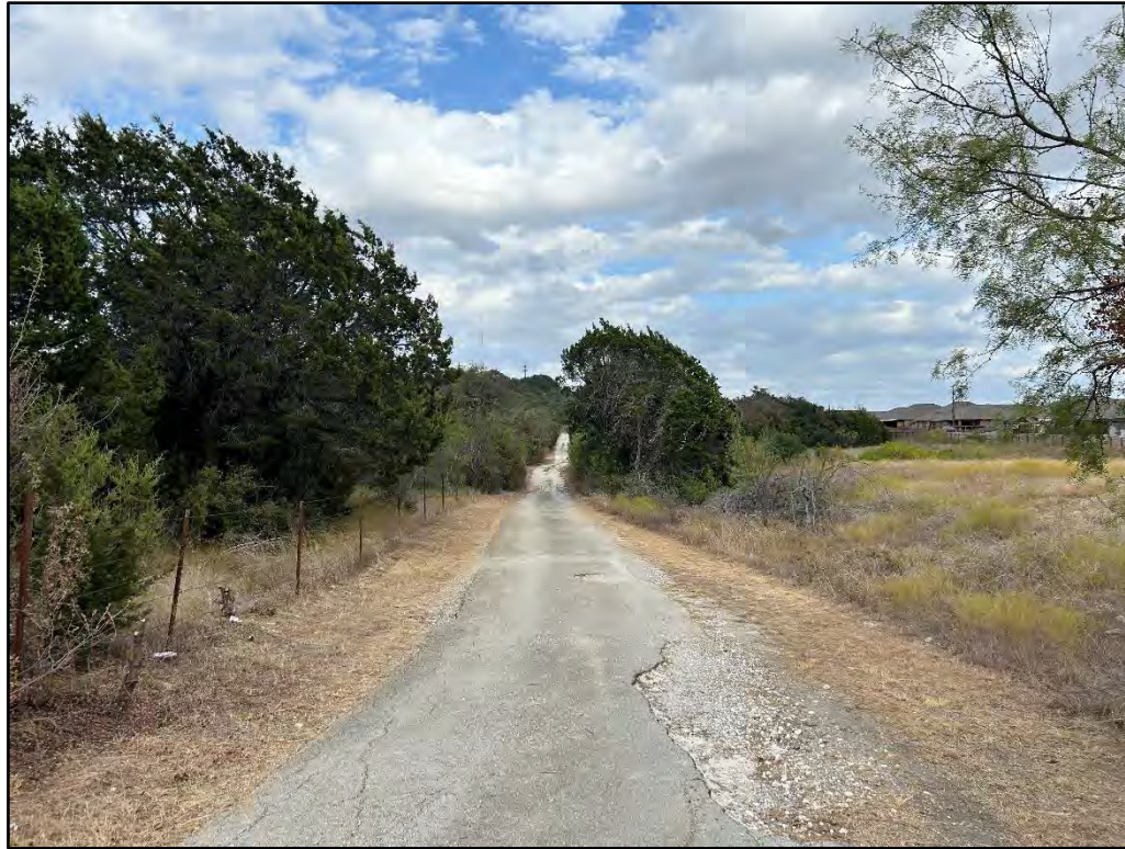
Tower Hill Lane – First section is old asphalt, then gravel, then rough cut road along the hillside
