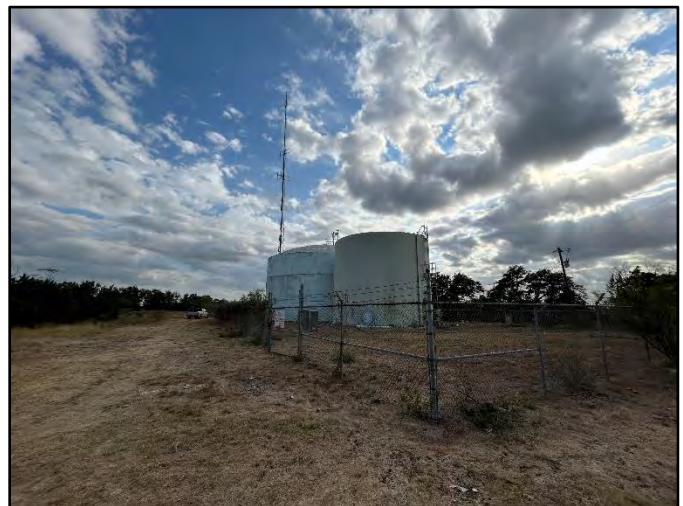
Existing Two Tanks/Location of New Tanks
