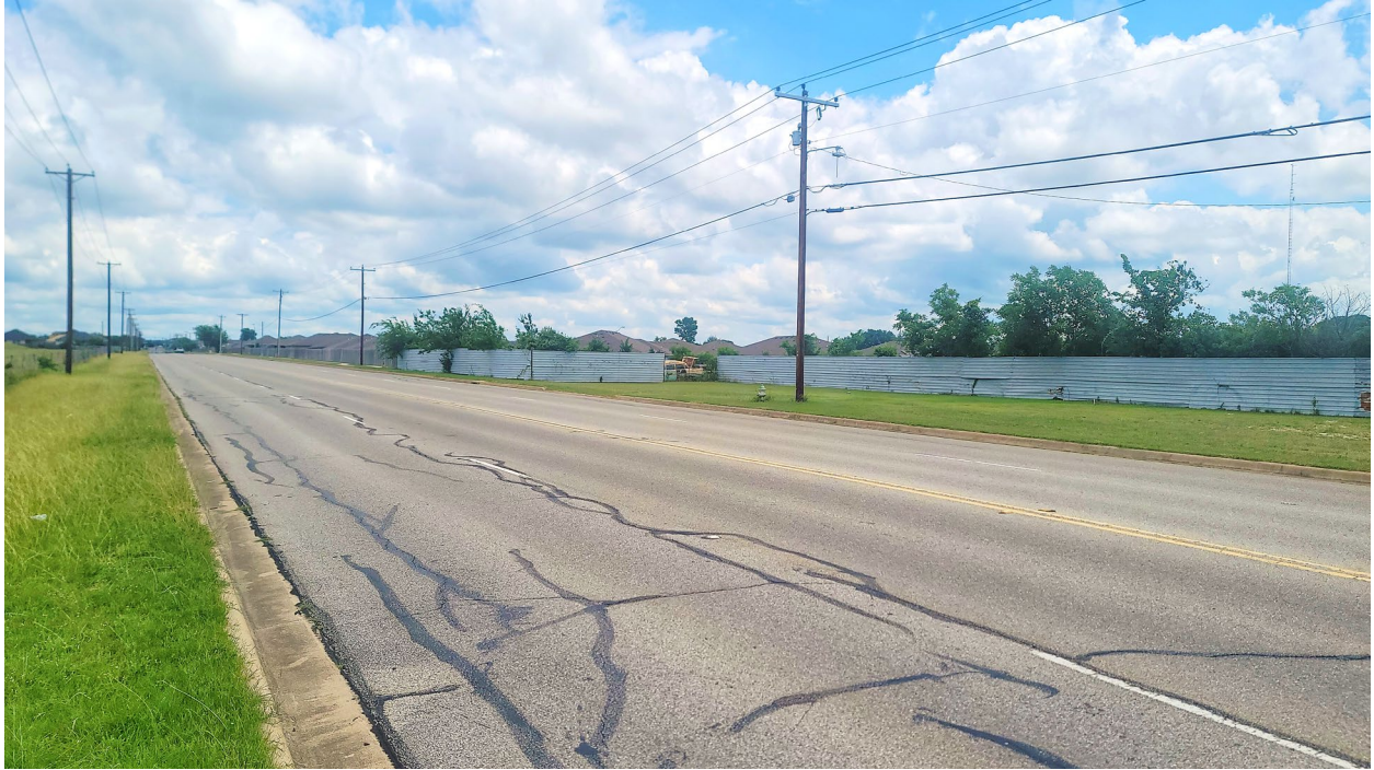
View facing north along N Roy Reynolds Drive:
