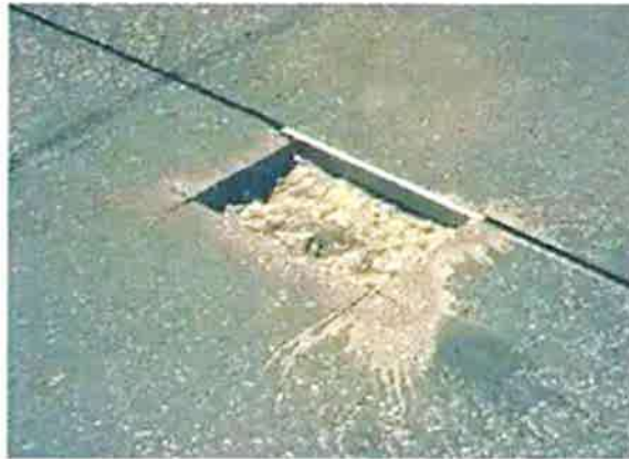
Figure 3-4 Compressible Insert. From UFC 3-270-01 (2018), for reference only.
