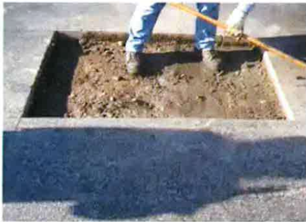
Figure 3-1 Damaged Pavement Removed by Sawing. From UFC 3-270-01 (2018), for reference only.
