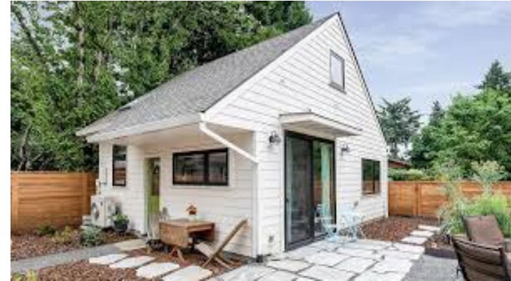
Tiny house on slab
