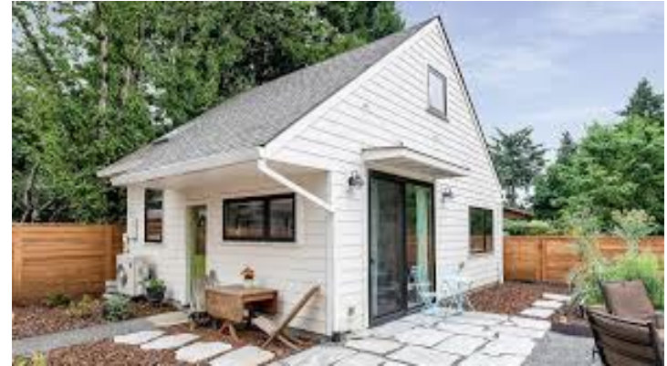
Tiny house on slab
